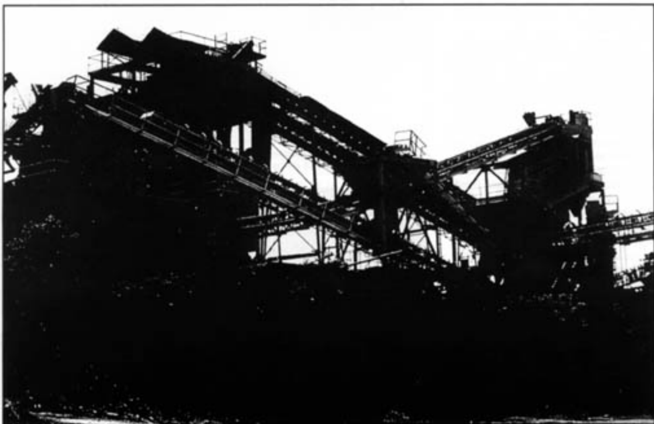
Balf Co.'s secondary plant (foreground) produces asphalt aggregate in a closed circuit with two 1560 Nordberg Omnicones, a Barmac vertical impactor and two 8 x 20 ft Nordberg screens fitted with Isenmann Flex-a-thon screens. A 100-ft screening tower can be seen in the background.
